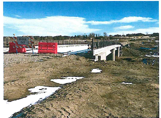
Scott Road Bridge
