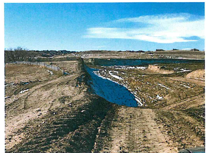
Village B Over Excavation
