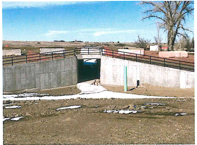
Scott Road Pedestrian Underpass
