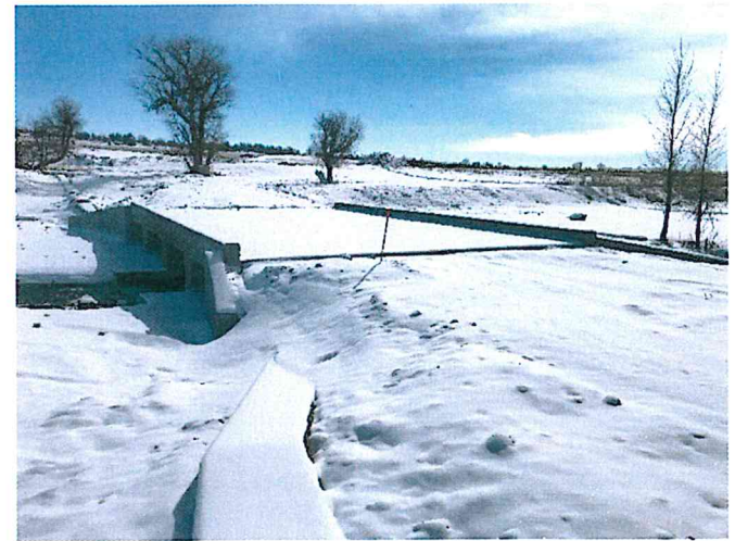
Low Flow Structure
