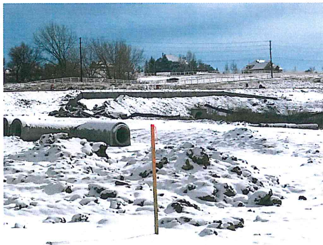
Retaining Wall at Drainage Crossing Parker Road
