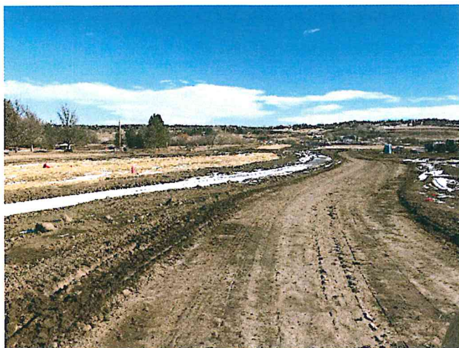
Village A Sidewalk from Pedestrian Underpass
