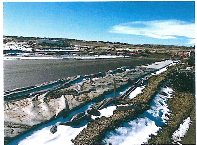
Village A Paving
